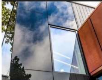
Aluminium windows adjacent glass cladding panels
