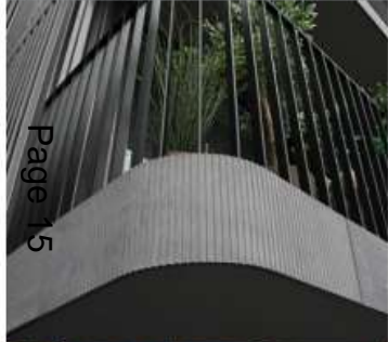
Metal balustrading adjacent GRC cladding panels
