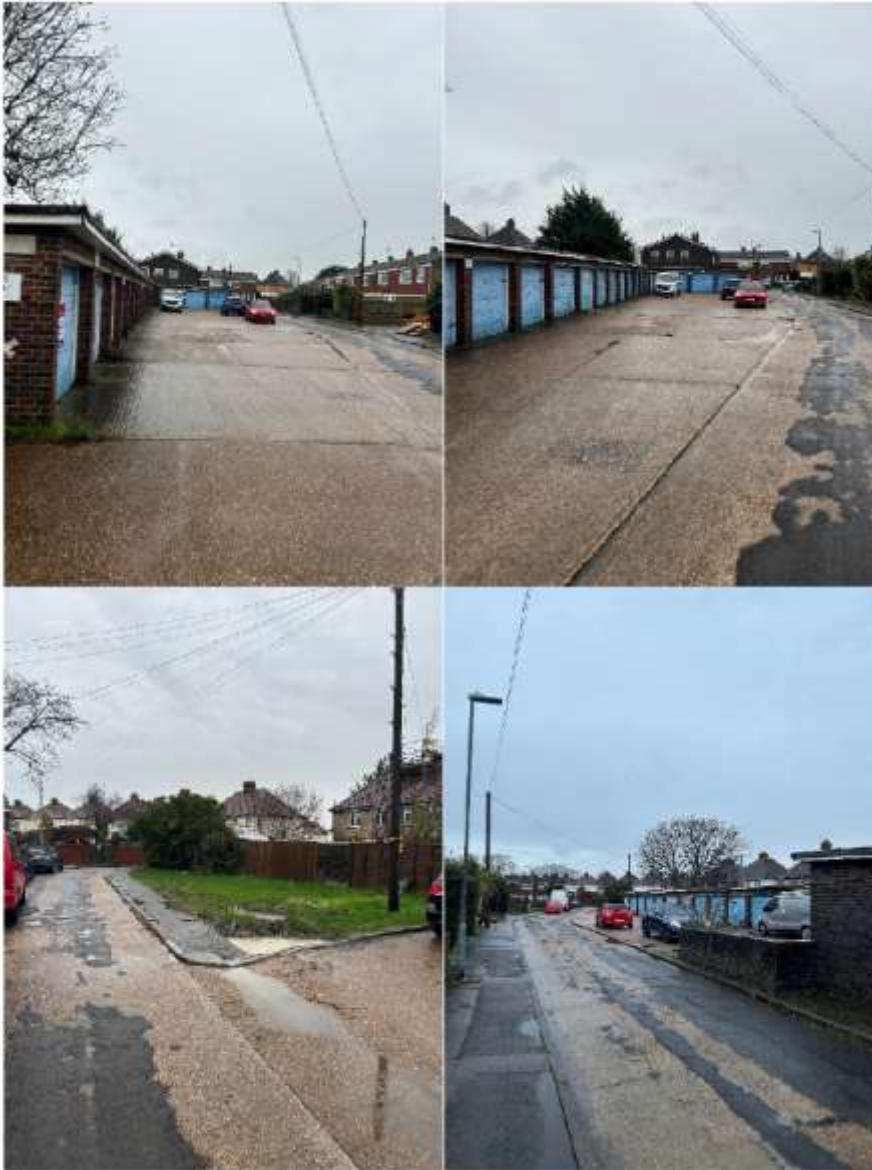
The existing garage block and grass verge.
