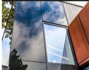
Aluminium windows adjacent glass cladding panels
