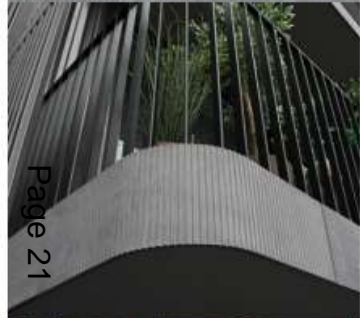
Metal balustrading adjacent GRC cladding panels
