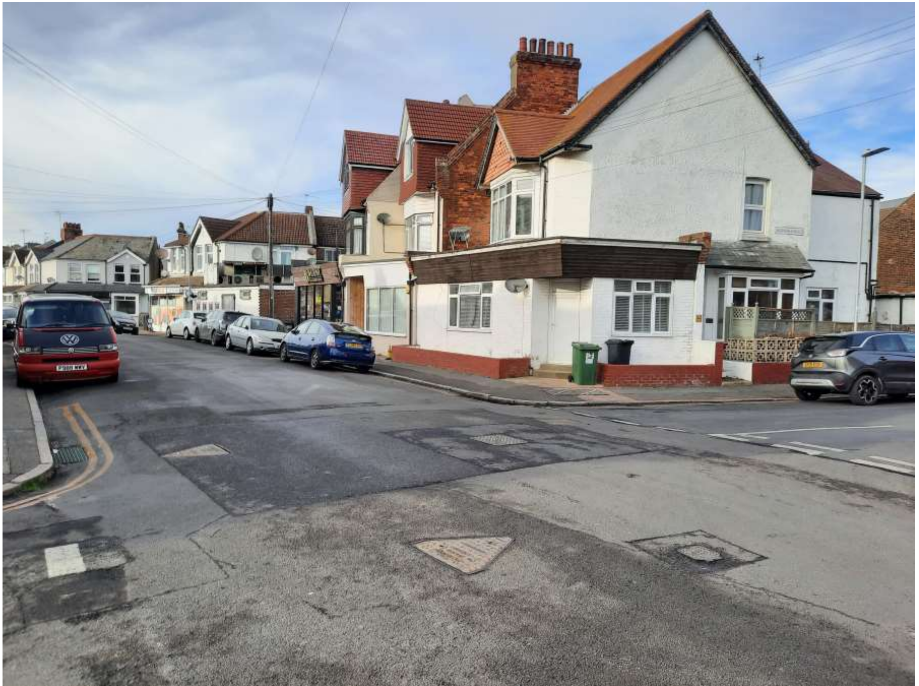
View from east – note adjoining converted shop
